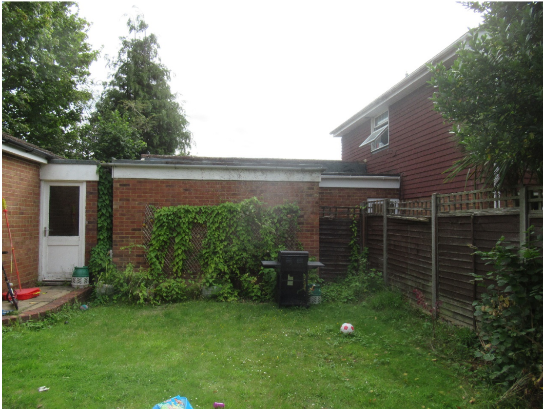
View of garage between No.6 & 8 Orchard Close from garden of No.6
